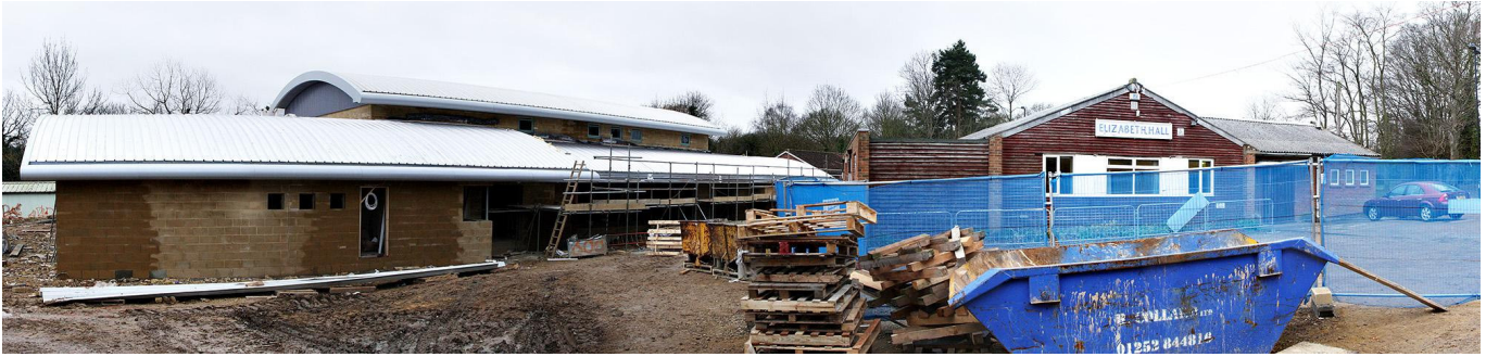
The new Elizabeth Hall is taking shape alongside the old.
